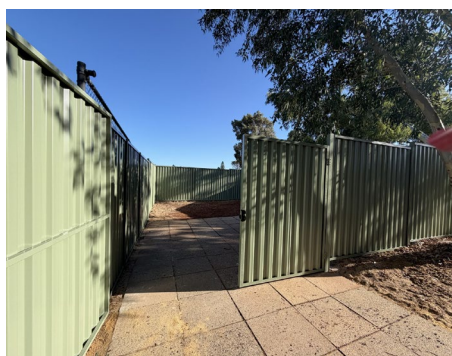
The completed bike shelter and secure fencing.
